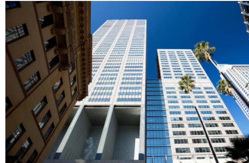
Governor Phillip Tower in heritage context
